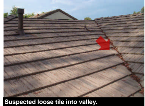
Suspected loose tile into valley.
