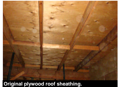
Original plywood roof sheathing.
