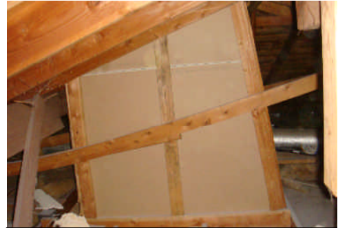
View of the skylight, lacking insulation.
