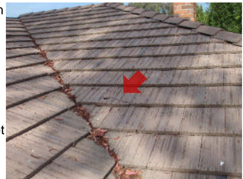
Suspected loose tile into valley.
