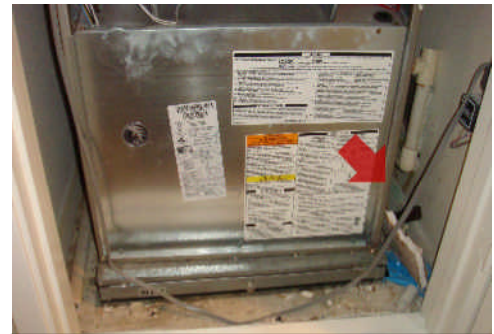
Remove all debris and abandoned pipes.
