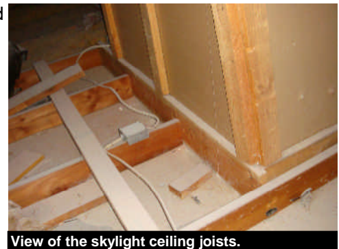
View of the skylight ceiling joists.
