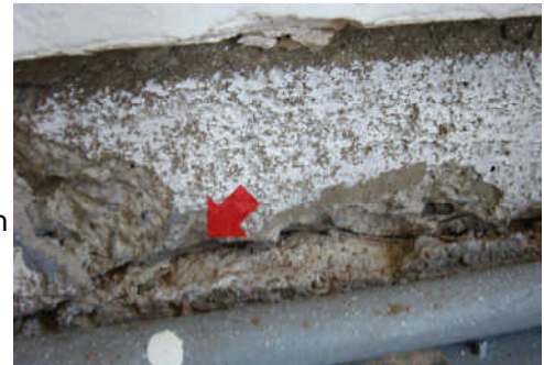
Garage right side foundation /slab.
