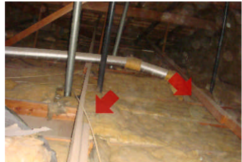
Wall ties are from left to right walls.
