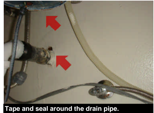
Tape and seal around the drain pipe.
